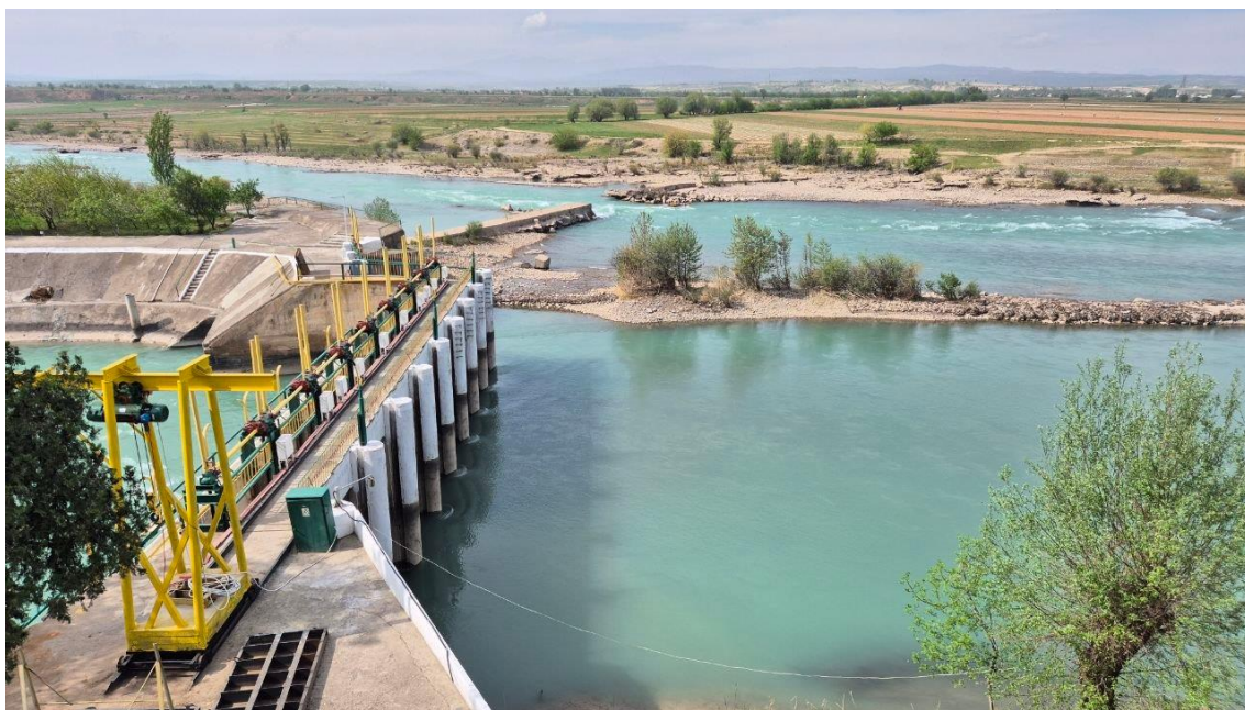
Headworks of Big Fergana Canal
