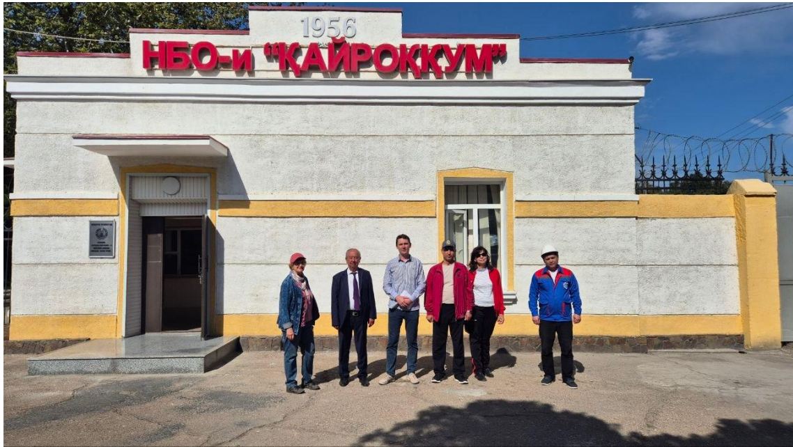
Building of Kayrakkum HPP
